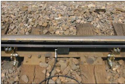
Lincoln wiper bar = open, clean ports
