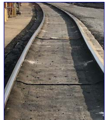
Spilltration® Husky PolyBack Track Mat 19 Months After Installation.
